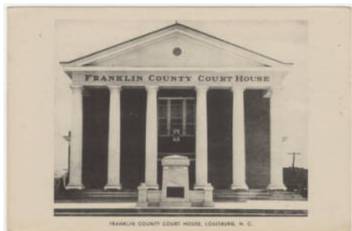
Franklin County Courthouse, Louisburg, NC
