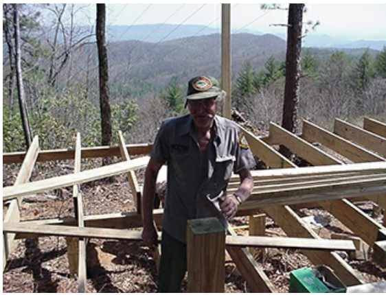
Park staff building a structure with a scenic view behind the work site, Gorges State Park. Photograph, April 11, 2001. North Carolina Division of Parks and Recreation.
