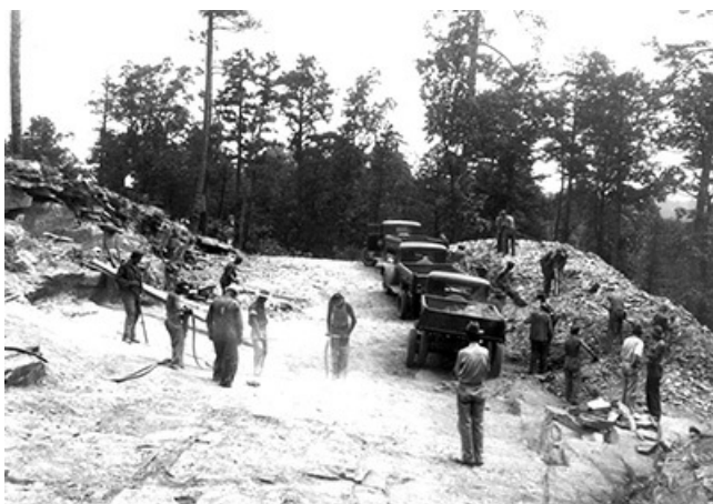
Workers in the Civilian Conservation Corps at the rock quarry during dam construction, ca. 1935-1942, at Hanging Rock State Park. Image from the collection of North Carolina State Parks.
