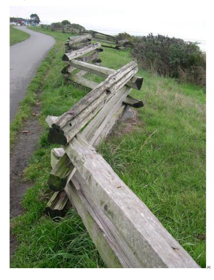
In a zigzag fence, the rails are laid "zagly" on top of each other, without posts.
