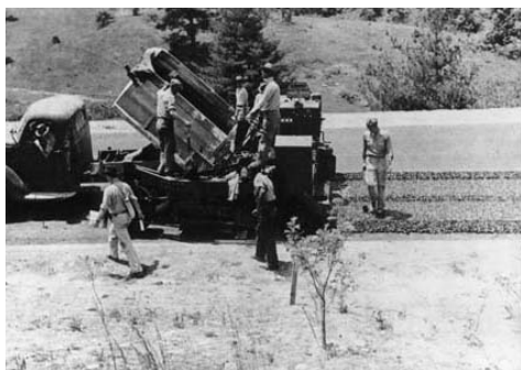
[2] Civilian Conservation Corp (CCC) workers paving a section of the Blue Ridge Parkway.
