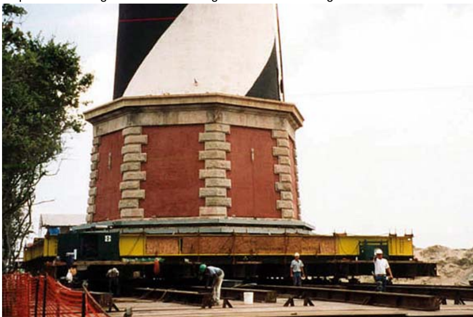
The lighthouse on tracks during its relocation.
