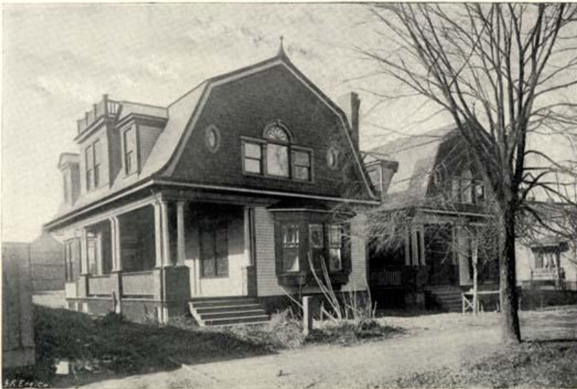
Fig. 29. Superintendent's House. Cost $1,500
