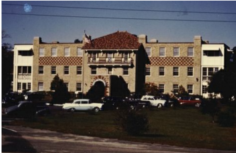
"Photograph of the front facade of the Babies Hospital, Wrightsville Beach." Image courtesy of the Historical Society of the Lower Cape
