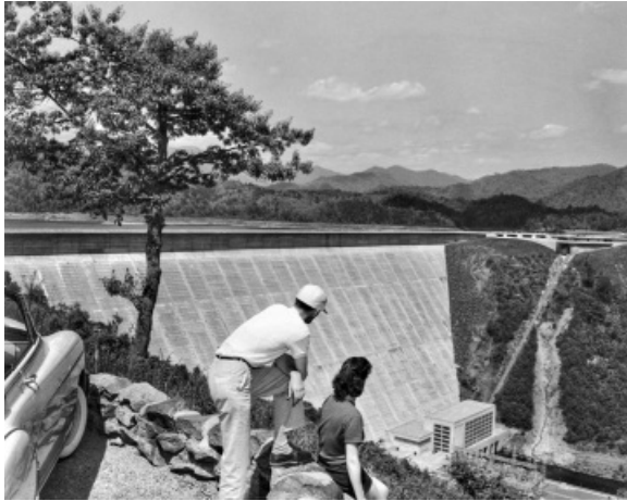
A view of the Fontana Dam and powerhouse, 1950s. North Carolina Collection, University of North Carolina at Chapel Hill Library.
