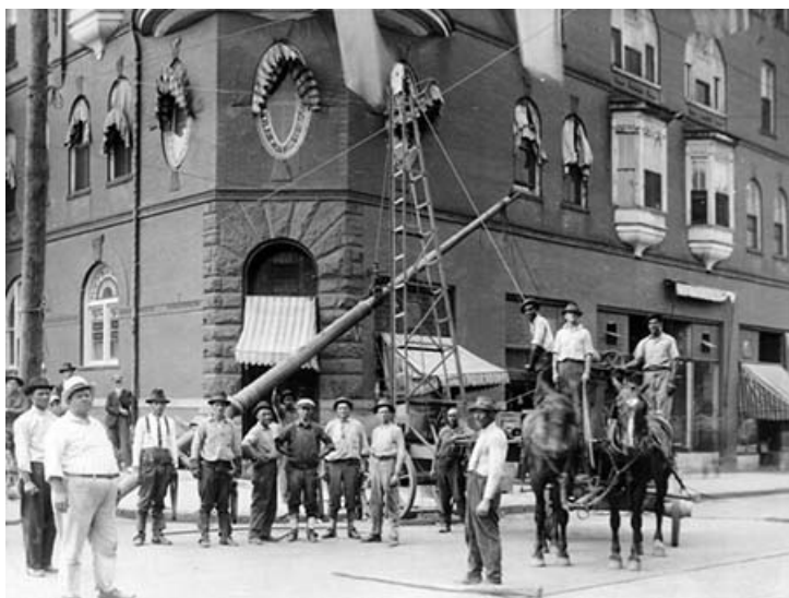
A Carolina Power and Light line crew seen posing for a photo at the corner of W. Martin and McDowell Streets in Raleigh on July 5, 1916 as they hoist up a light pole with a team of horses. From the CP&L Collection, State Archives of North Carolina. Used courtesy of the N.C. Department of Natural and Cultural Resources.
