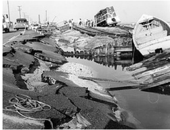
Damage from a 1960 NC hurricane. Image courtesy of the State
