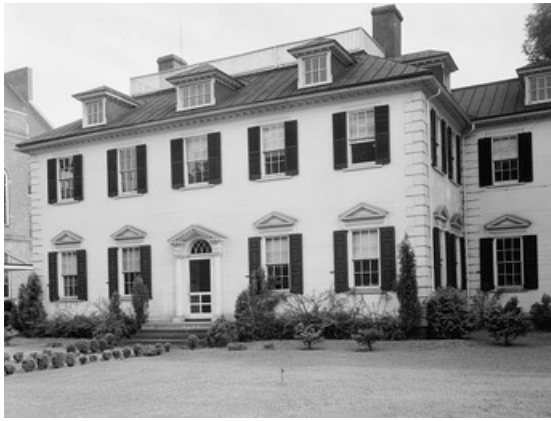
Frances Benjamin Johnston. Photograph of the John Wright Stanly House, New Bern, 1936. Image from the Library of Congress Carnegie Survey of the Architecture of the South.
