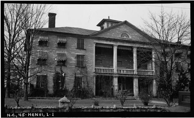
Library of Congress. "Historic American Buildings Survey, Stewart Rogers, Photographer February 20 1934 EAST ELEVATION (FRONT). - Judson College, Third Avenue & West Flemming Street, Hendersonville, Henderson County, NC, Women's College."
