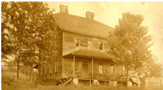
Mourne Rouge, Montfort Stokes' house near Wilkesboro, circa 1907-1929. It was destroyed by fire in 1971.
