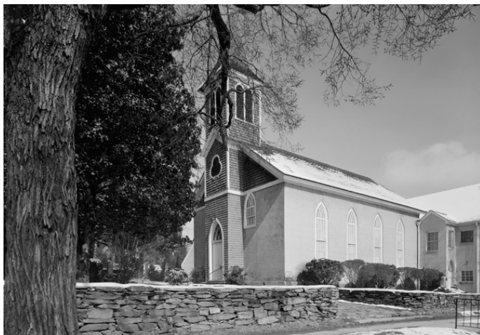
Photograph of the Hillsborough Presbyterian Church, Hillsborough, NC. From the Historic American Buildings Survey, Library of Congress Prints & Photographs Online.
